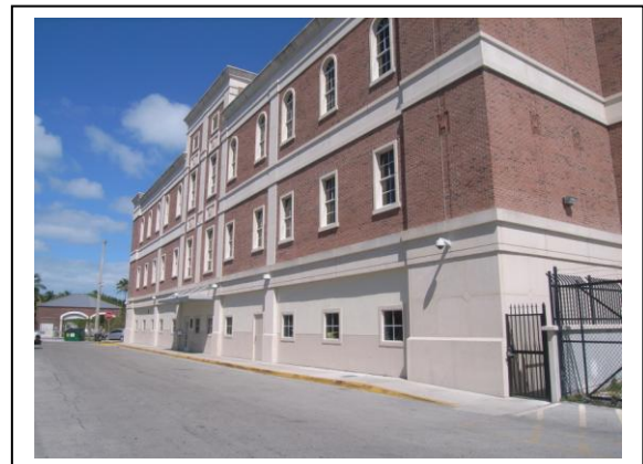
Rear – Entrance to Drug Court on 1 st Floor on Thomas Street
