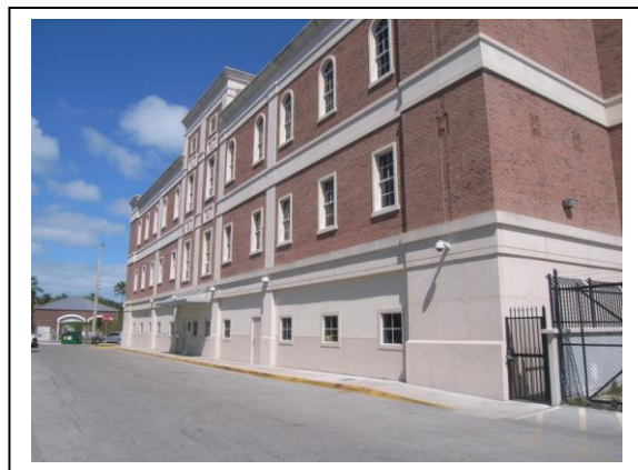
Rear – Entrance to Drug Court on 1 st Floor on Thomas Street
